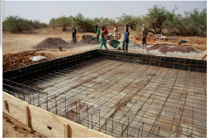
Building of a concrete reservoir to hold water for the elephants
