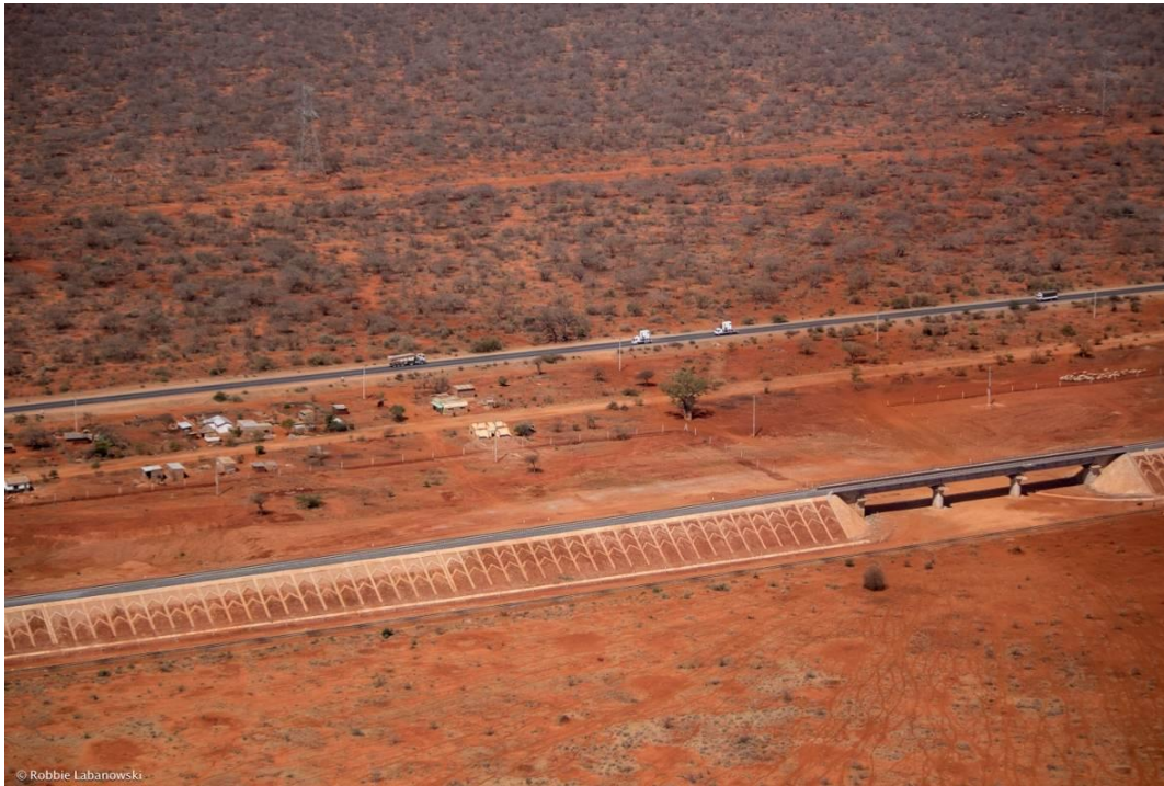
Plate 1a: Illegal Human settlement near an official Ndara corridor underpass at DK125
