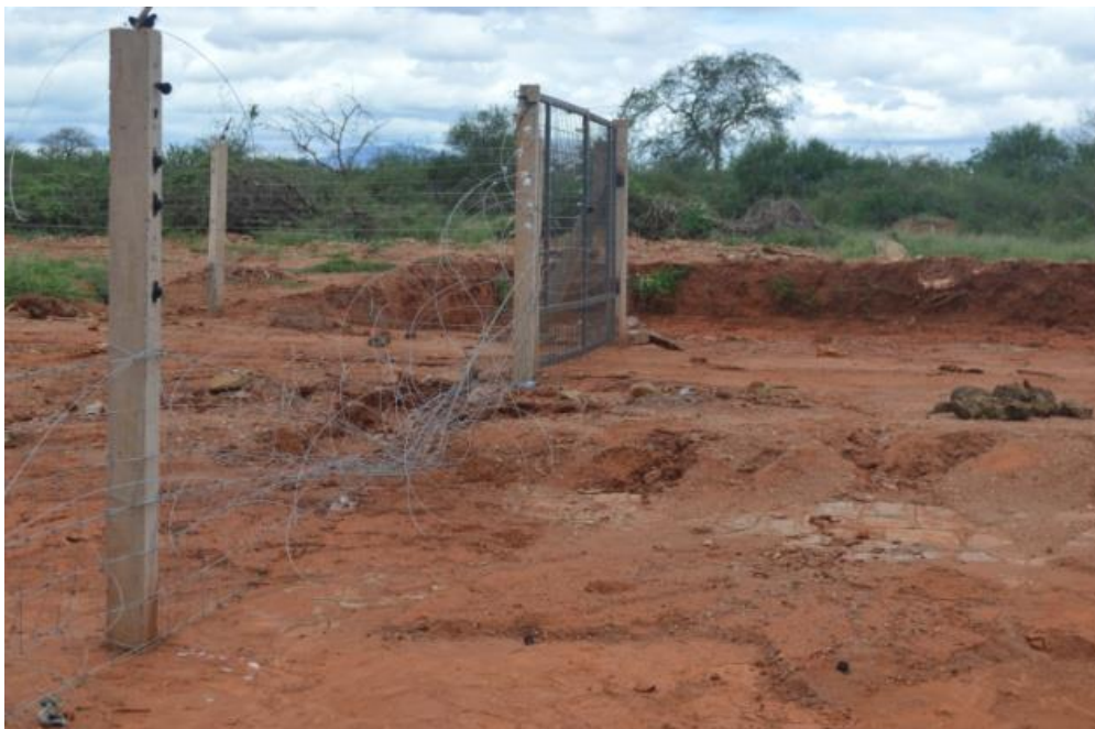
Plate 3a & 3b: Trapped elephants inside the SGR fence and breakages by elephants creating a high risk for collision between elephants and the SGR train. Photo Credit: Tsavo Trust and KWS
