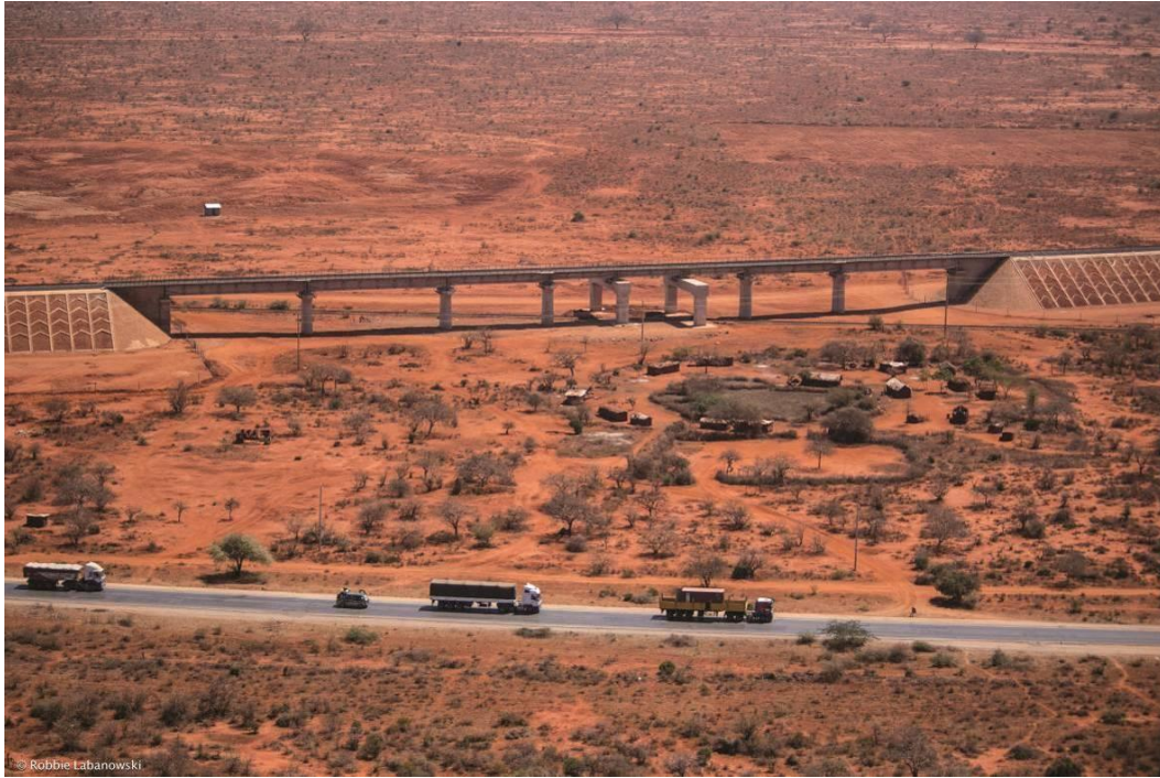
Plates 1b: Recent illegal human settlement at the Maungu SGR and old railway crossing, at DK118, that is highly utilised by wildlife. These settlements will inevitably suffer from human-wildlife conflict and should be moved before they become more permanent.
